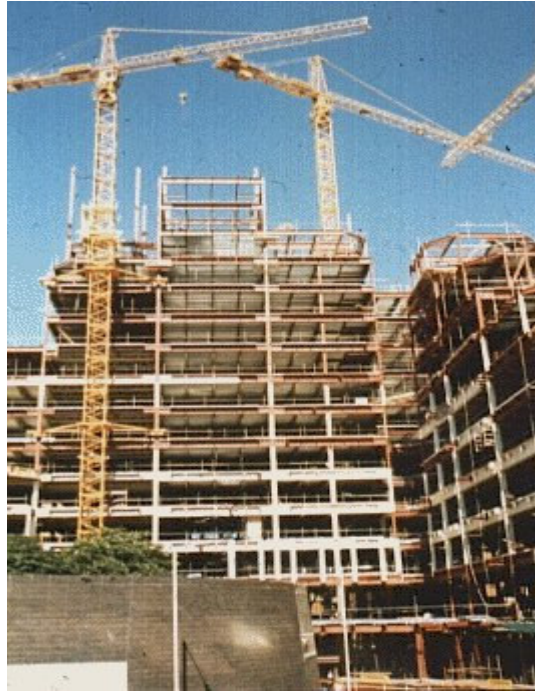
Picture 1 : Typical composite multi-storey steel-framed building during construction - a commercial building in London.
