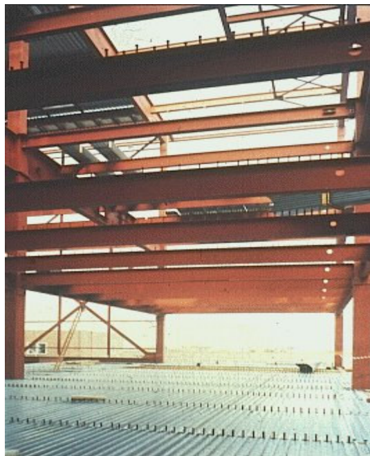
Picture 2 : Typical composite multi-storey steel-framed building during execution - a factory building for the car industry in Germany.
